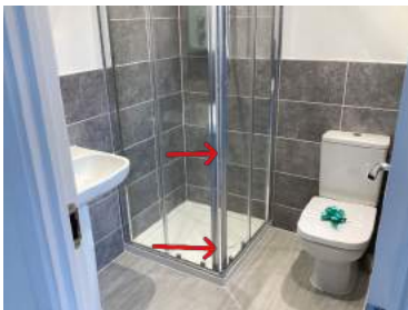
EN SUITE 2 Shower enclosure doors not joining together correctly
