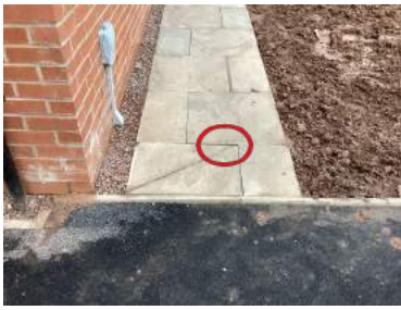
GARDEN Paving slabs uneven
