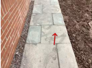
GARDEN Paving slab cracked
