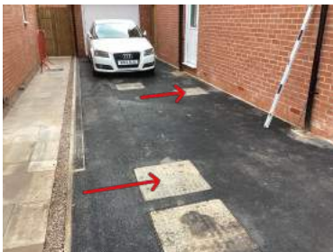
DRIVEWAY Inspection chamber lids not fitted correctly
