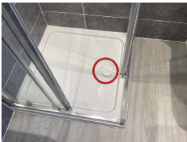
EN SUITE 2 Incorrect shower tray drain cover fitted
