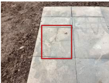
GARDEN Paving slab cracked
