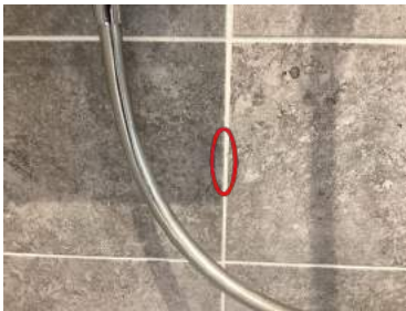
EN SUITE 2 Various holes to grouting in shower enclosure and corner RHS toilet
