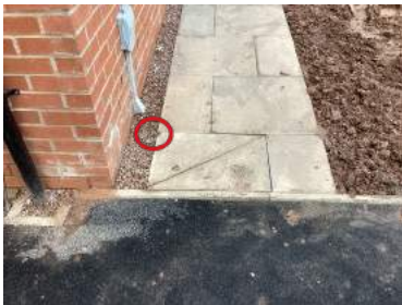
GARDEN Paving slab chipped
