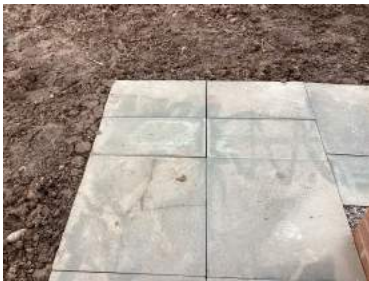
GARDEN Paving slabs loose and not tight together
