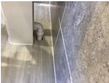
EN SUITE 2 Inadequate finish to flooring behind pedestal
